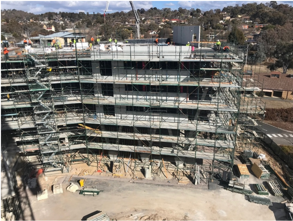
Building C Level 4 suspended slab being formed, steel reinforcement and stressing ready for pouring.
