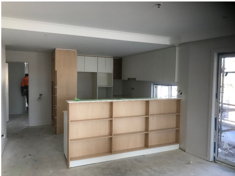
Kitchen, apartment 47, Building A ground floor.
