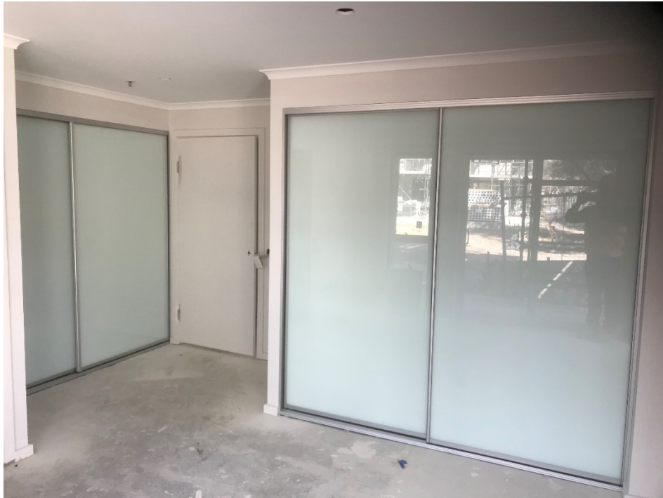
Main bedroom, apartment 51, Building A ground floor.
