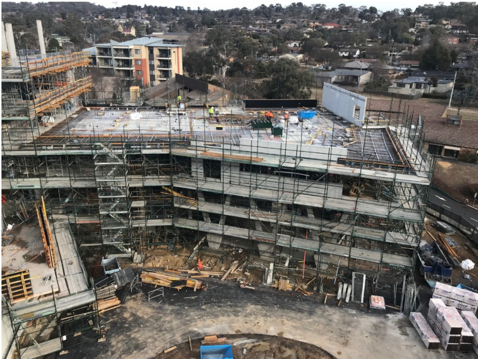
Building C Level 2 suspended deck formed, steel reinforcement and stressing installed.
