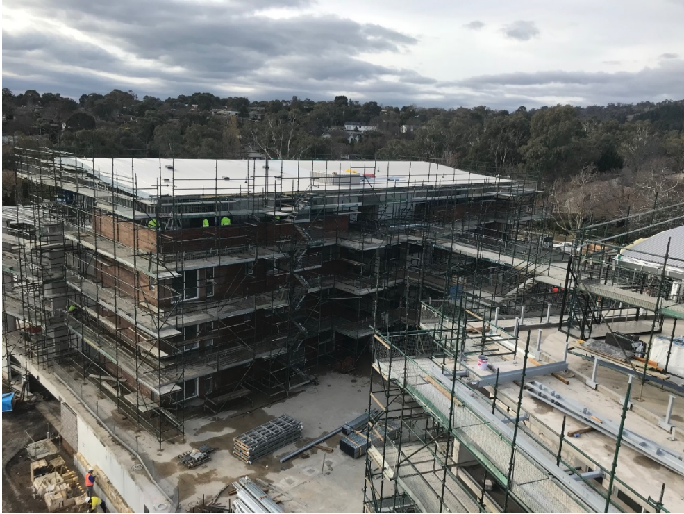
South-west elevation of Building A, roof installed, brickwork complete to Level 3.
